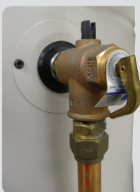
TPR position - top of cylinder
