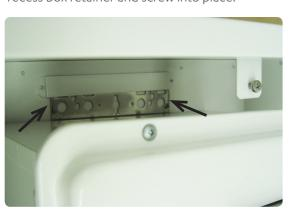
4. Lower the EF24 mounting bracket keyhole over the centre screw. Fit additional screws.
