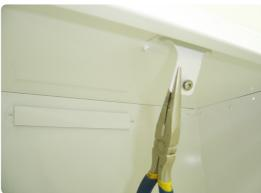
3. Slide the EF24 top mounting bracket under the recess box retainer and screw into place.
