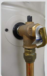
TPR position - top of cylinder
