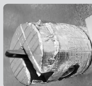
Insulated TPR valves will look like the image below
