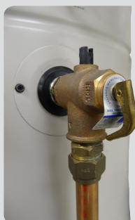
TPR position - top of cylinder
